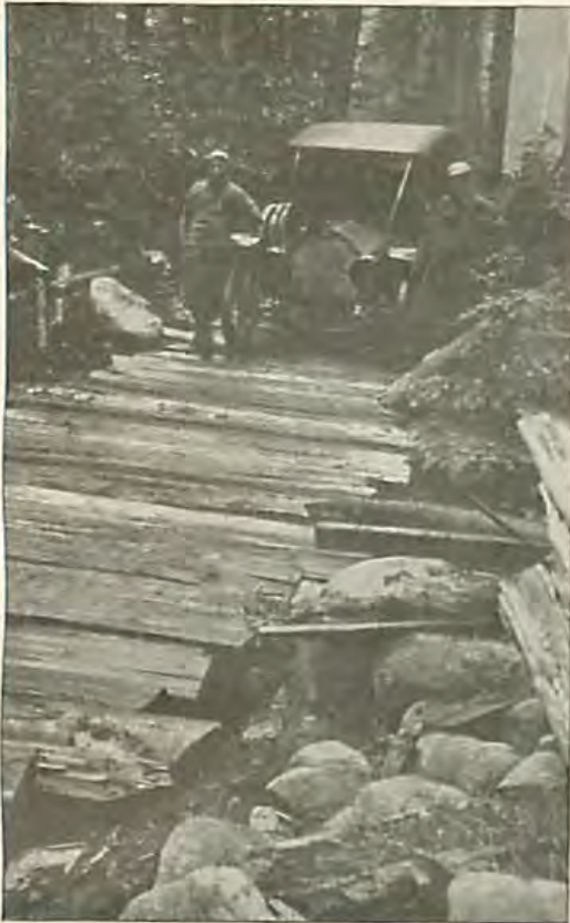
CORDUROY ROAD BETWEEN PORTLAND AND ASTORIA, OREGON. THIS WAS THE FIRST MOTOR CAR TO TRAVERSE THIS ROAD.
